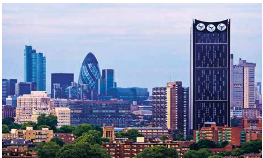
1-2-nji surat. Ýel generatoryny beýik binanyň üstki böleginde ýerleşdirmek usuly (London ş. ýaşayuş jaýy) Photo No. 1-2. Method of placing a wind generator on the roof of a high-rise building (apartment building in London)
